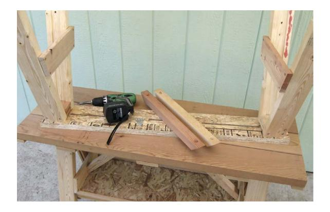
With the leg assemblies attached it is time to attach each diagonal braces with 2 (two)  $\#8\ X\ 1\frac{1}{2}$ " washer head screws.
