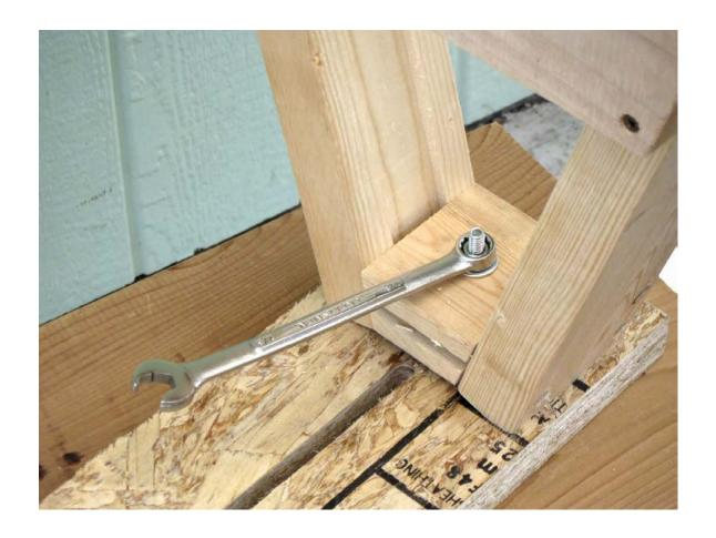
... and place a 5/16" flat washer and a 5/16" hex nut over the ends of each bolt and tighten securely with a wrench.
