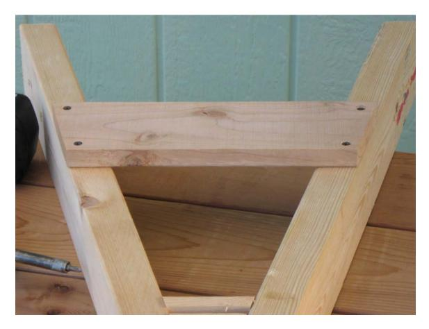
"Square up" each lower brace and position it so the two ends of the lower brace are flush and even with the outside faces of the legs as shown here. Then fasten each lower brace to legs with four  $\#8 \times 1\frac{1}{2}$ " screws. The photo above shows how it should look when each lower brace is attached to a leg assembly.
