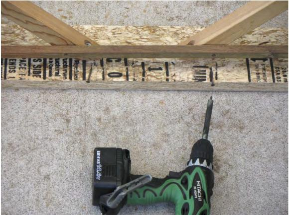
Here the #8 X 1<sup>1</sup>/<sub>2</sub>" screws are about to be attached to the diagonal brace through the pre-drilled holes in the **CLAMP-it**<sup>TM</sup>. When this is done the **CLAMP-it**<sup>TM</sup> is ready for use.
