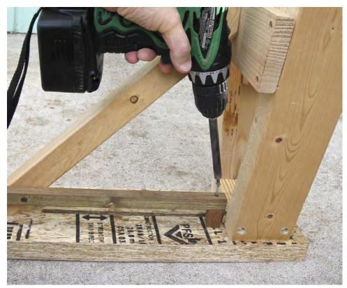
The **CLAMP-it<sup>™</sup>** has been placed with a standoff under each end so that the #8 X 2½" screws will go through the hole pre-drilled in each end of the **CLAMP-it<sup>™</sup>** and through the centered holes that go along the lengths of the standoffs. The **CLAMP-it<sup>™</sup>**s have also been positioned to ensure that the #8 X 1½" screws will be drilled into the diagonal braces. (see photo above)
