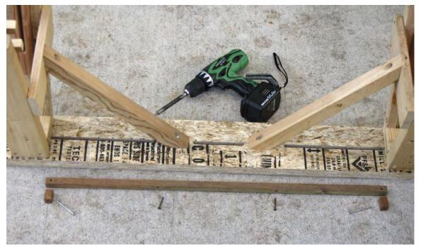
Here a **LEVEL-it**<sup>®</sup> is lying upside down in preparation for the **CLAMP-it**<sup>™</sup> to be mounted to the underside of the **LEVEL-it**<sup>®</sup> top. There is a **CLAMP-it**<sup>™</sup> with two standoffs, 2-#8 X 1½" screws and 2-#8 X 2½" screws. In this instance self-drilling or auger tip screws are being used so no pre-drilling is necessary.
