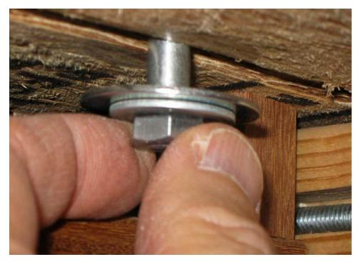
With the **TOP-it<sup>™</sup>** placed on top of the **LEVEL-it**<sup>®</sup> thread each bolt up through a slot in the **LEVEL-it**<sup>®</sup> top as shown here and hand tighten each into a Tee-nut.
